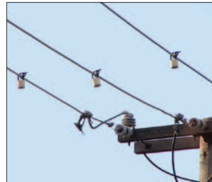
CRDs provide fault indication in a low-voltage application.
