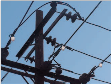
BTRI_IR Fault Indicators installed on an overhead system.
