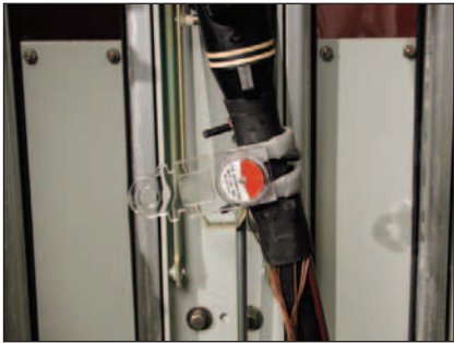
The Manual Reset Fault Indicator is an excellent troubleshooting tool for both overhead and underground applications.
